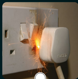
Loose connections or components within a socket or device.
